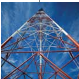
Radio base station
