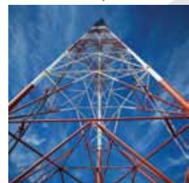
Radio base station
